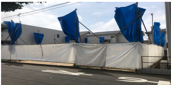
Temporary enclosure on 11 May 2020
