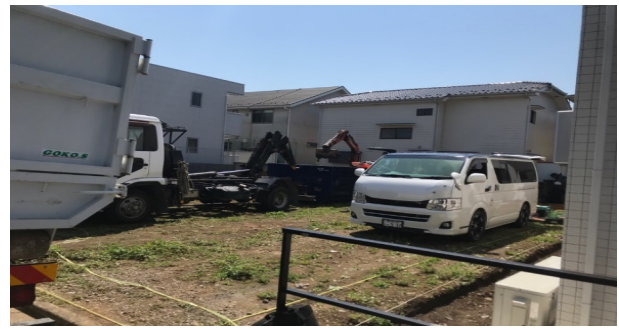
Well digging on 25 April 2020
