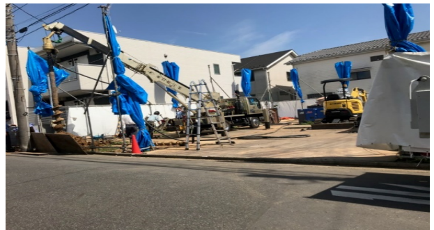
Start of H steel driving underground on 15 April 2020
